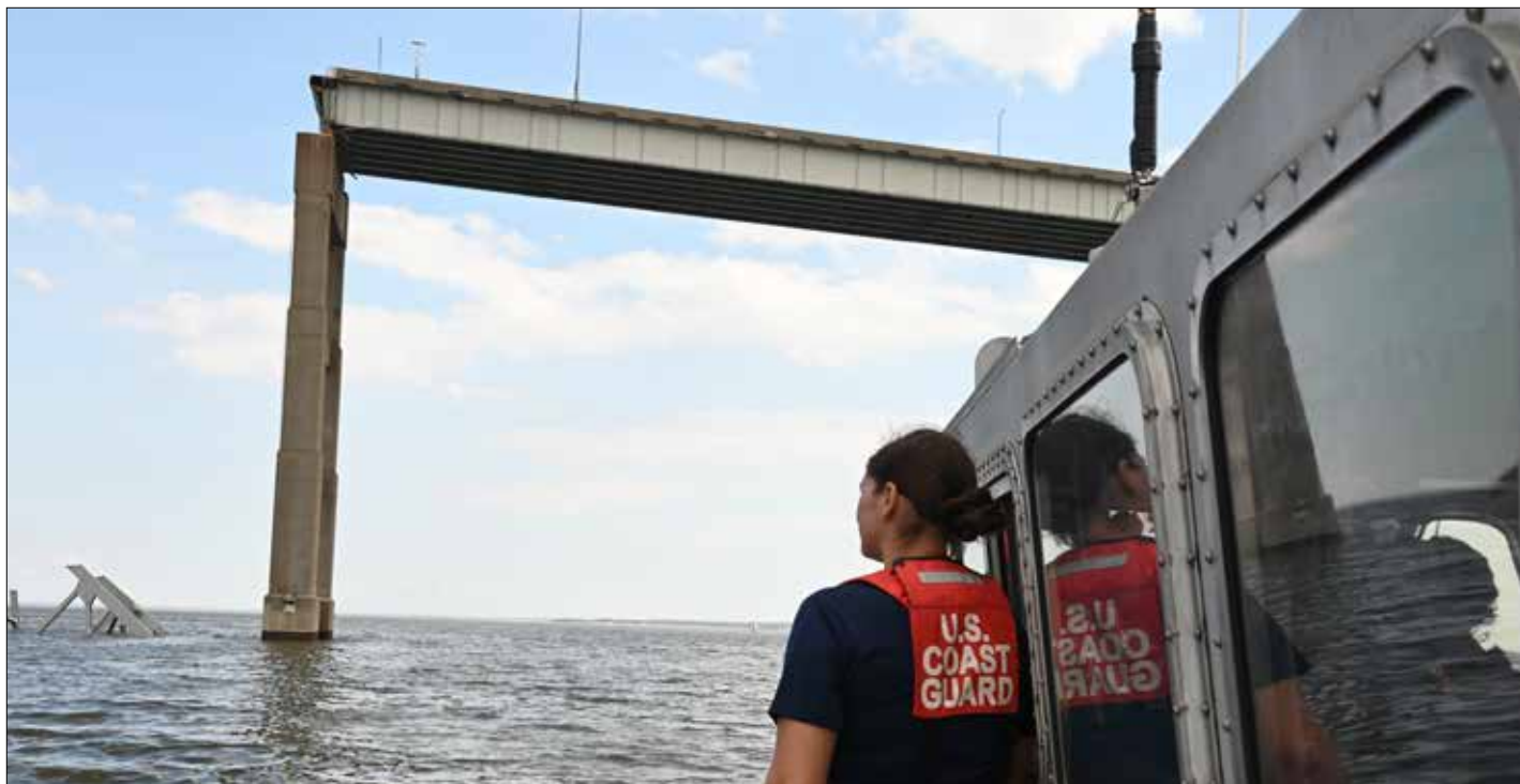
Petty Officer Third Class Amber Boguslawski, a boatswain's mate from U.S. Coast Guard Station Hatteras Inlet, North Carolina, looks out at the wreckage of the Key Bridge collapse in Baltimore, Maryland, April 10, 2024. The Key Bridge Response 2024 Unified Command priorities are to ensure the safety of the public and responders, account for missing persons, safely restore transportation. (Key Bridge Response 2024 Unified Command photo by Coast Guard Petty Officer First Class Lauren Steenson)
